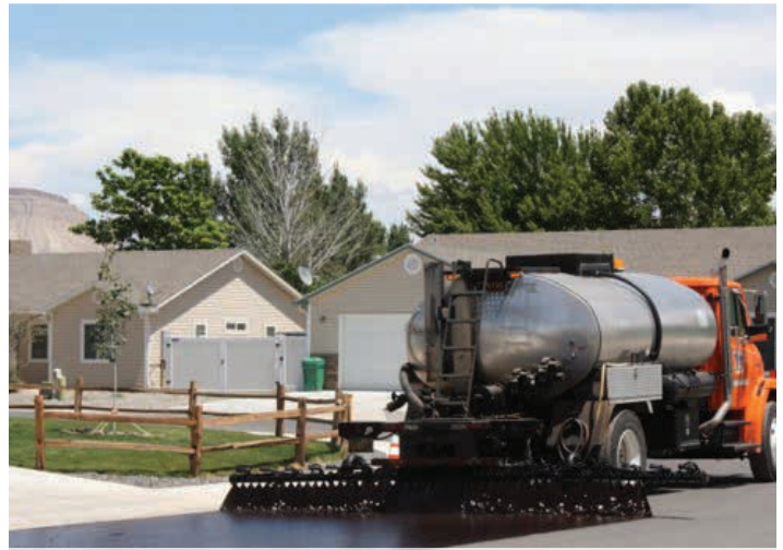
Application of polymer-modified chip seal emulsion using BASF latex
